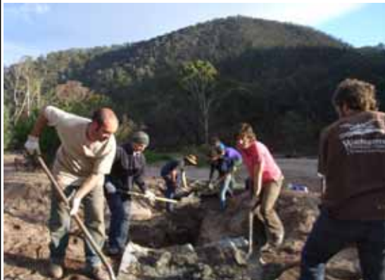
Mixing 1 cubic metre of cement by hand.
