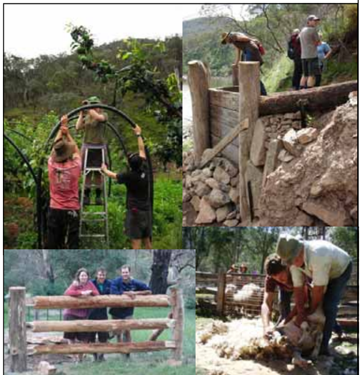
Clockwise from top left: Netting the fruit forest, checking out the solid construction of the new fox platform, Gaz and Richard shear a sheep, the new post and rail entrance fence.
