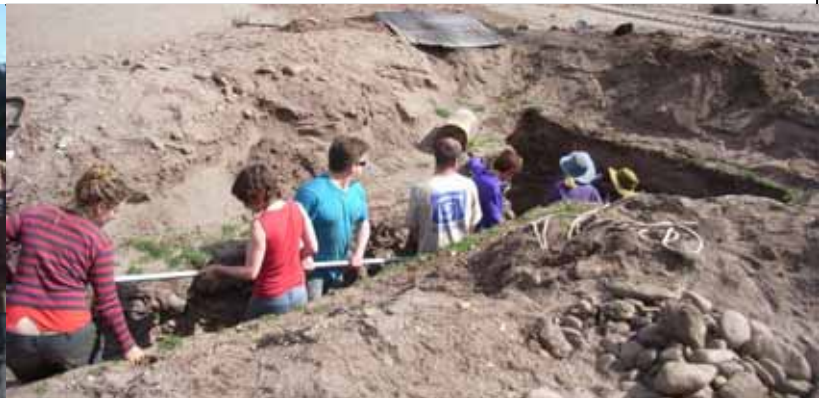
Laying in the anchor rod
